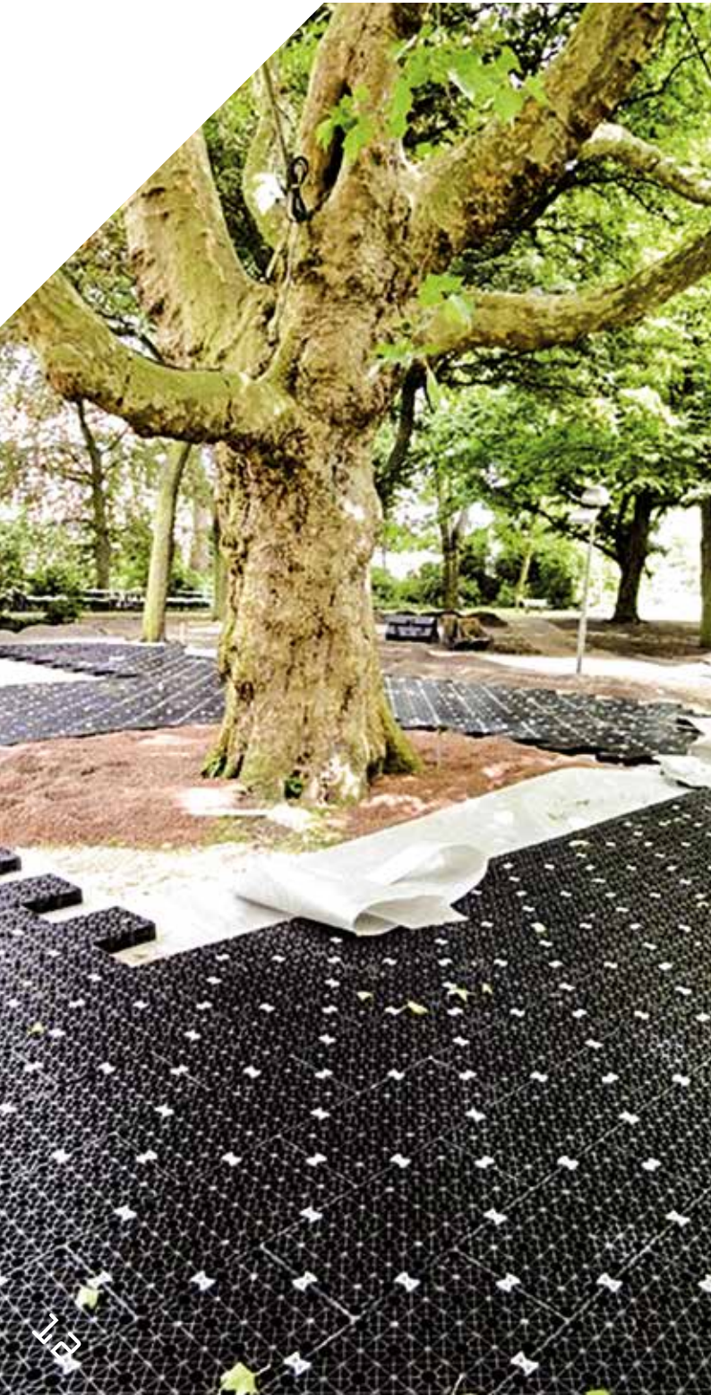
< Tolhuistuin Amsterdam. The Permavoid subbase is used under a semi-paved surface to protect the roots of a monumental London Plane tree when transforming a former garden into an event area.
