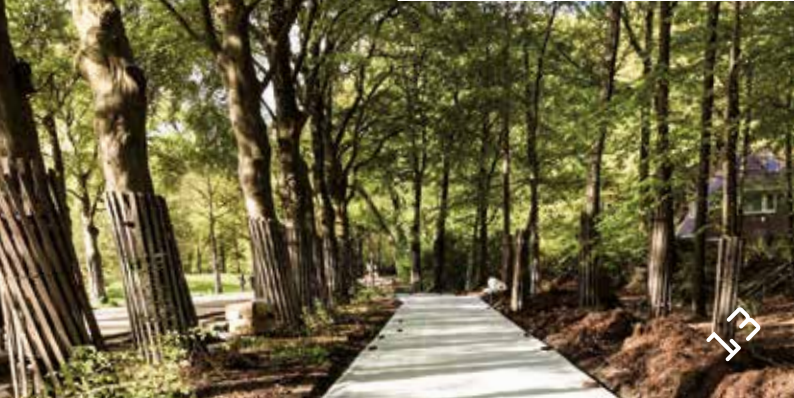
> Epe Heerdeweg. A floating bicycle path. For bicycle paths through existing green infrastructure, the shallow application and the lightweight construction are of particular importance in order to prevent damage to the rooted profile.
